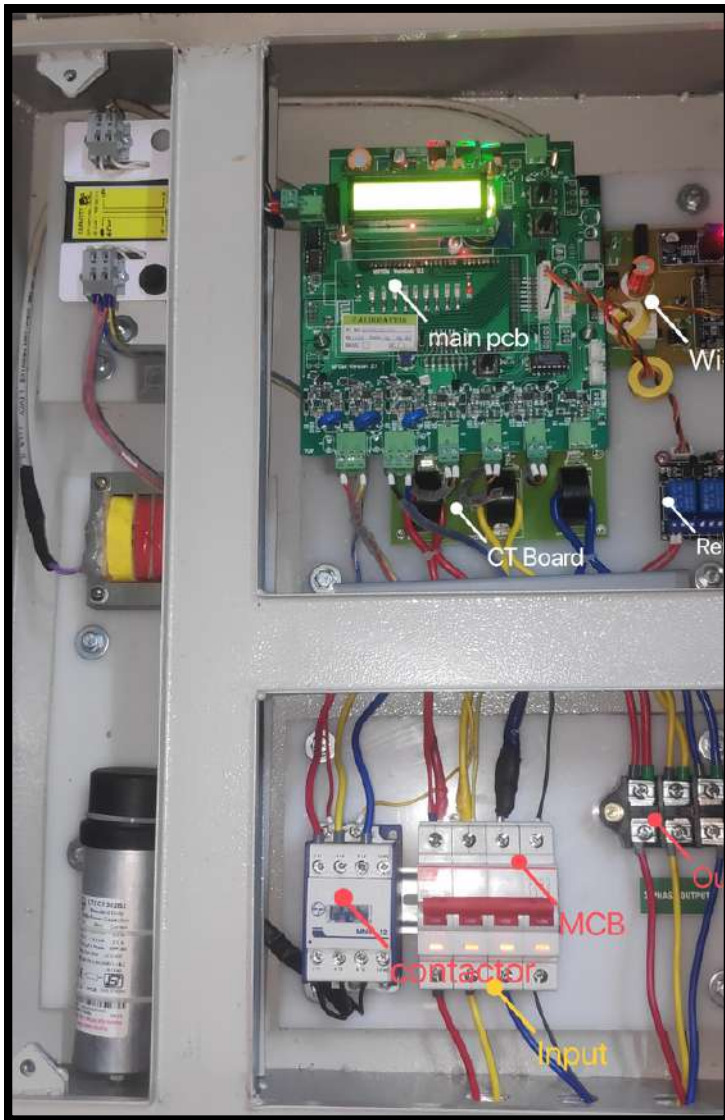
DelSmartIoT - DRCU Hardwares Single Step and Multi Step
