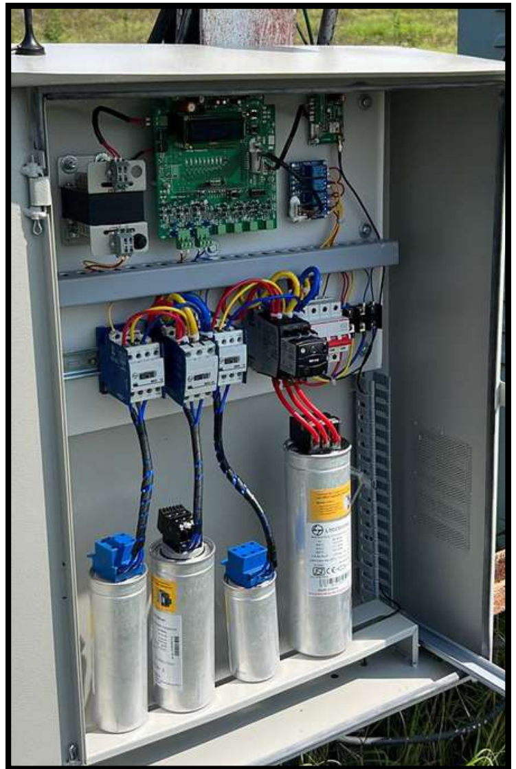
DelSmartIoT - DRCU Hardwares Single Step and Multi Step
